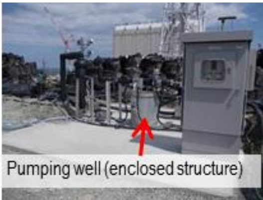
Figure 1: Pumping well for groundwater bypassing
