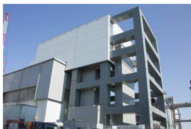
Equipment for fuel removal
