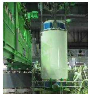
Storage of removed fuel
