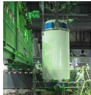
Storage of removed fuel
