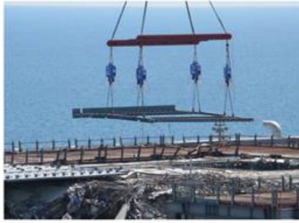
Installing shields on the operating floor
