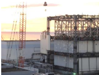
Dismantling of wall panels
