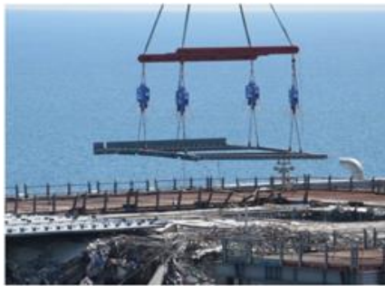
Installing shields on the operating floor
