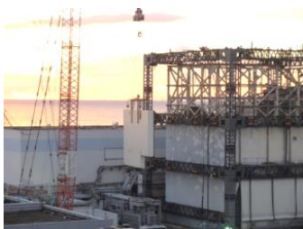
Dismantling of wall panels
