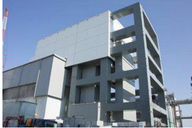
Equipment for fuel removal
