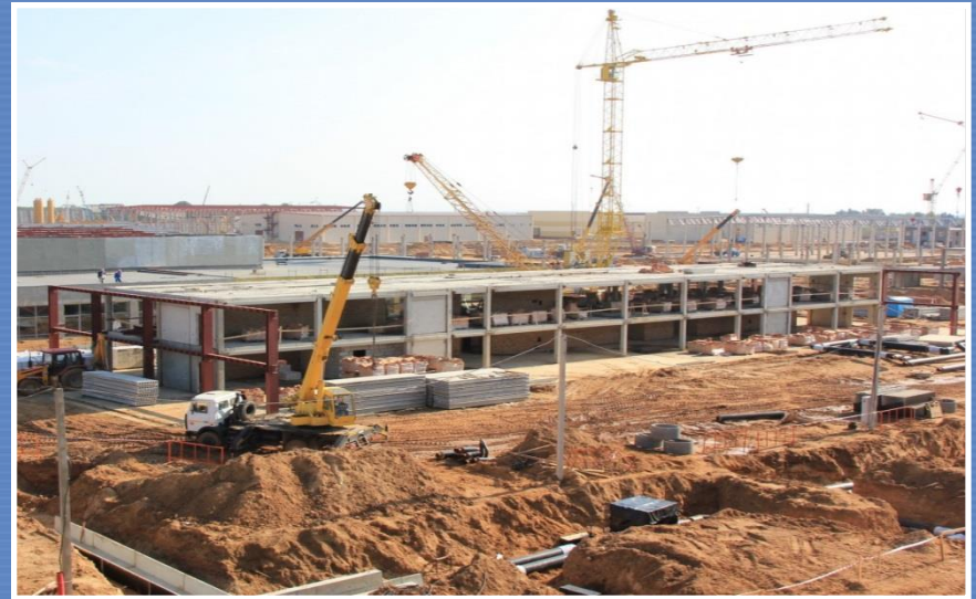
Preparatory work at the Ostrovets site, March 2013
