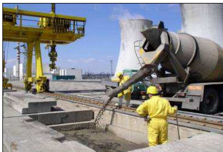
Fig. 8.3 Closing a full vault with concrete
