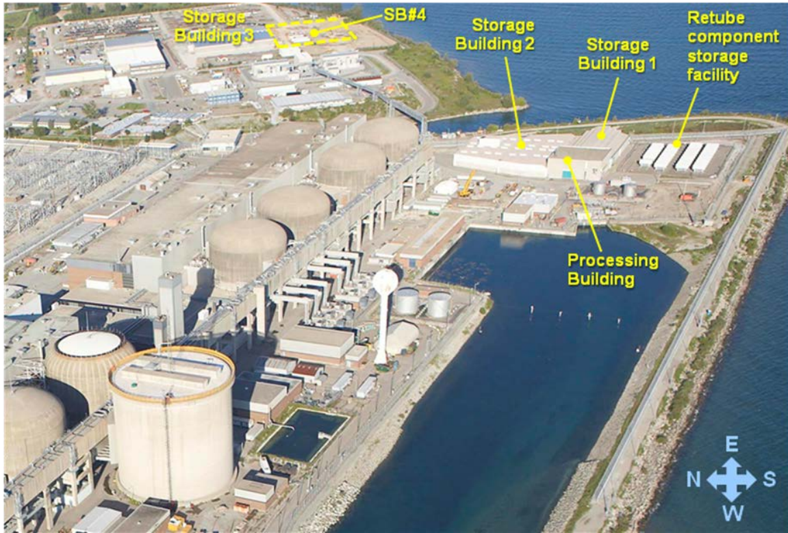
Figure 4.5: PWF I (Processing Building, storage buildings 1 and 2 and Retube Components Storage Building) and PWF II (Storage Building 3 and future storage building 4) area
