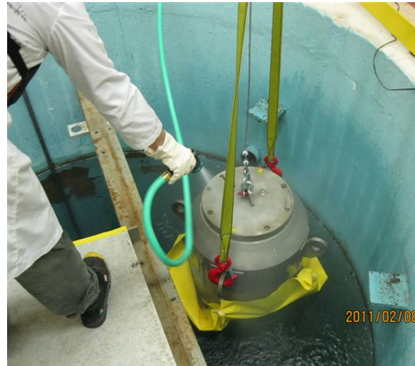
Figure 7.7: Removal of highly enriched uranium core shipping flask from reactor pool
