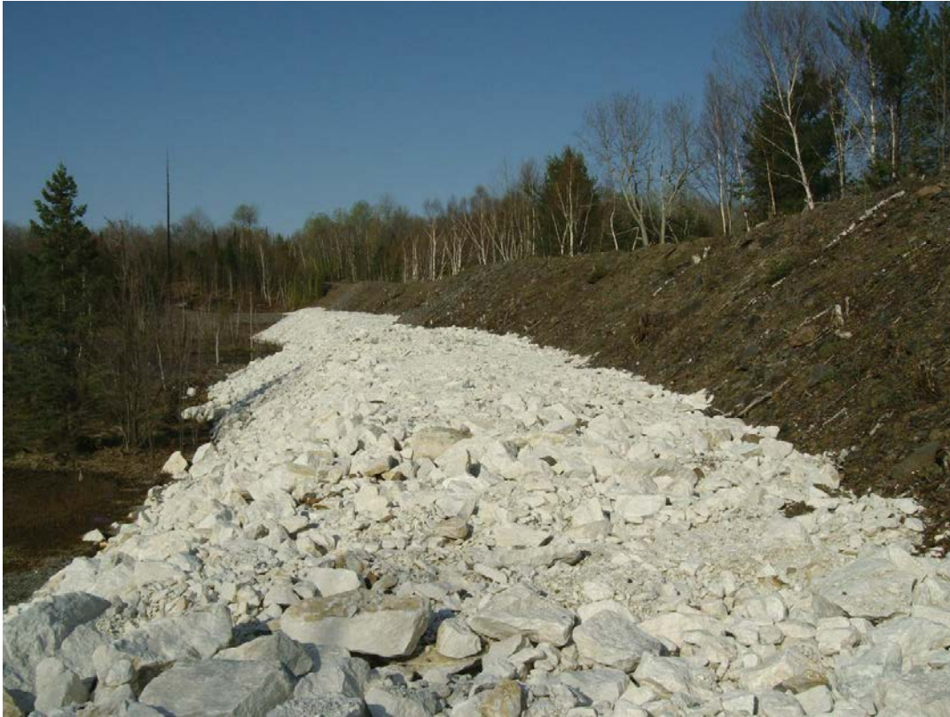
Figure 8.8: Main tailings dam, Dyno mine site
