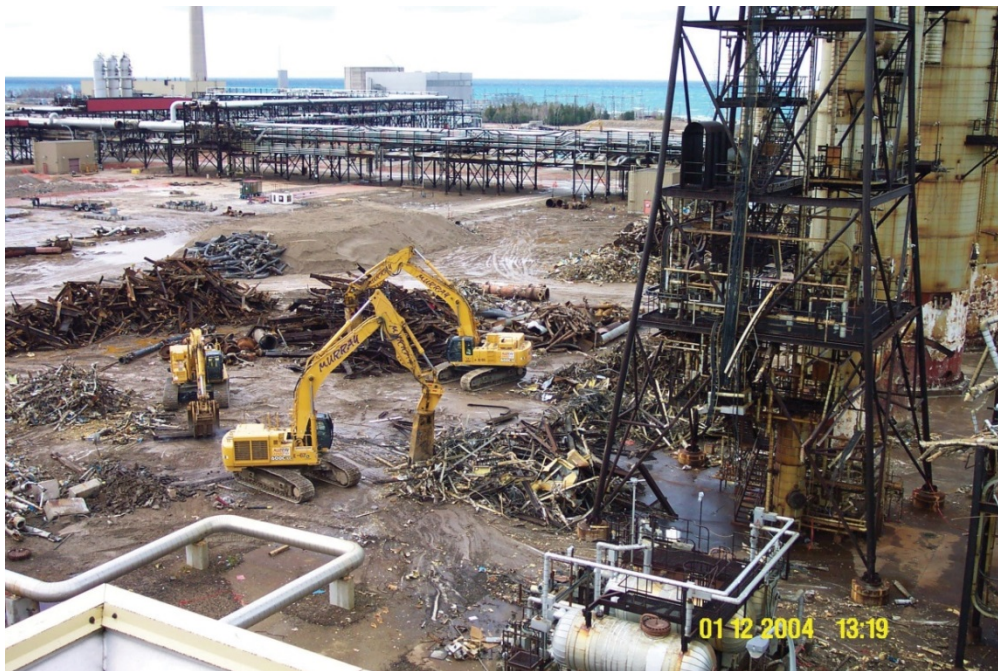
Figure 7.5: Demolition of the BHWP site
