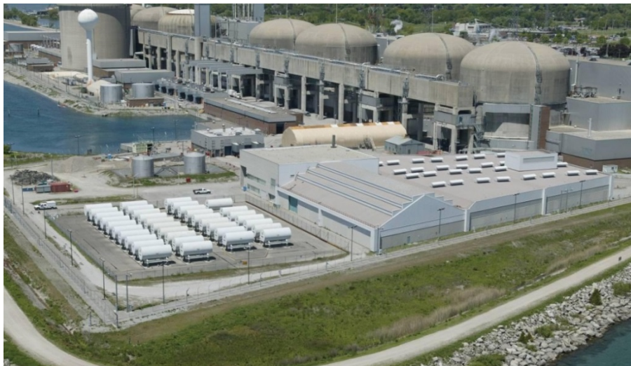
Figure 5.1: Pickering WMF, with RCSA (left) and spent fuel dry storage area (right)
