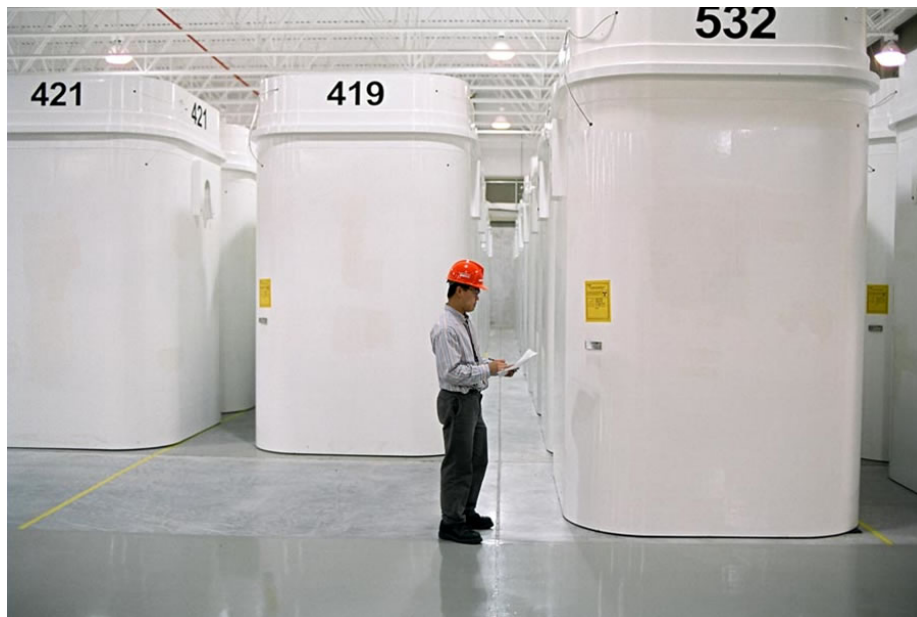
Figure 4.4: Dry storage containers at an OPG waste management facility
