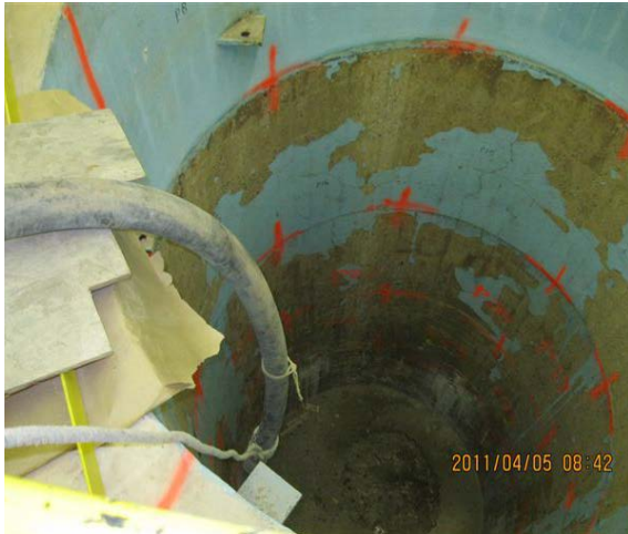
Figure 7.8: Backfilling pool with concrete
