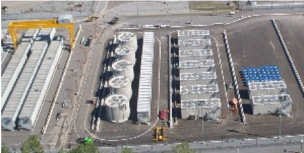
Figure 5.3: Gentilly-2 Solid Radioactive Waste Management Facility
