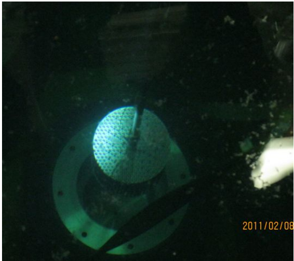
Figure 7.6: Removal of highly enriched uranium core from reactor container
