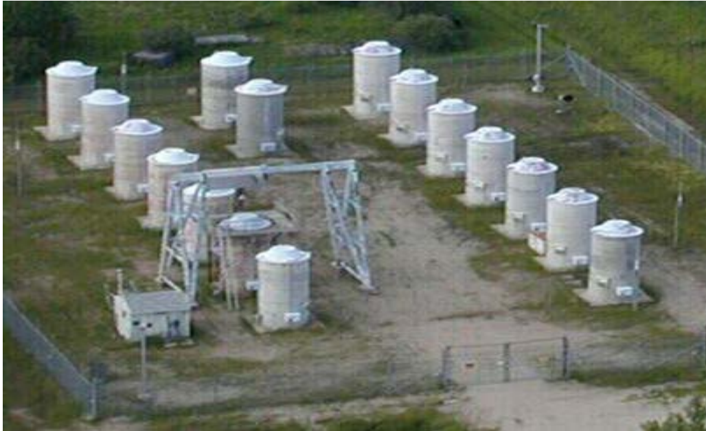
Figure 4.11: Whiteshell Laboratories Concrete Canister Storage Facility
