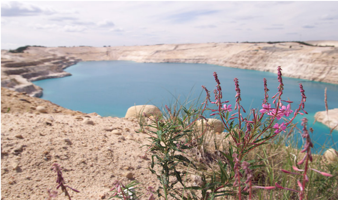
Figure 6.1: Deilmann Tailings Management Facility at Key Lake
