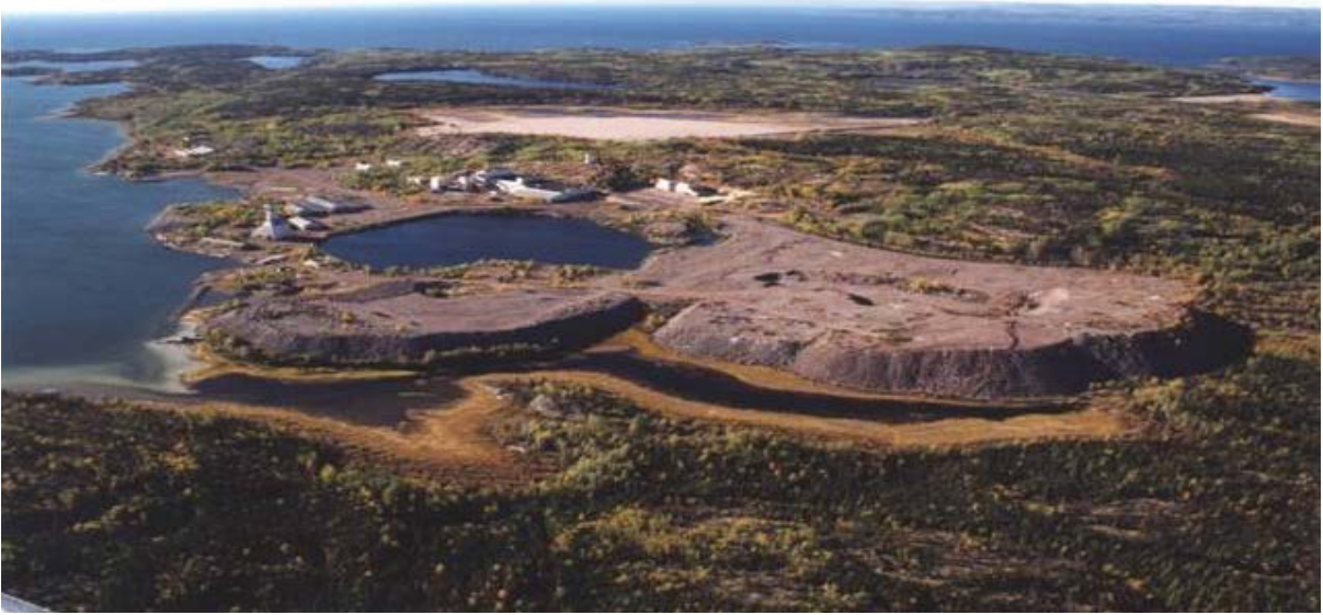
Figure 8.3: Before completion of CNSC order
