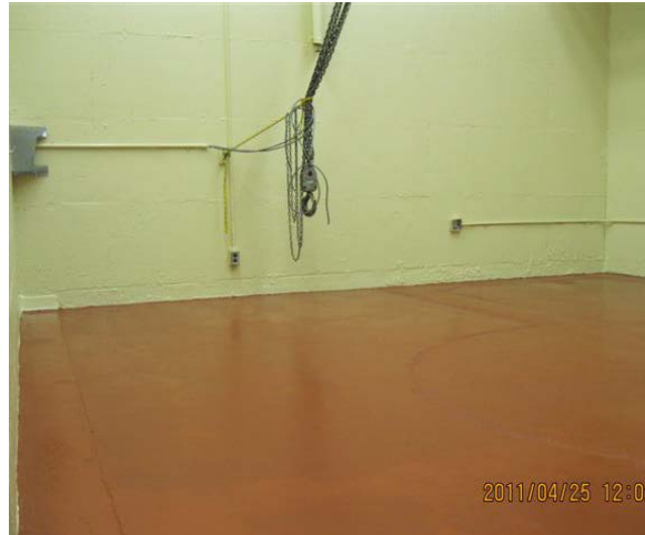
Figure 7.9: Filled and painted former reactor room
