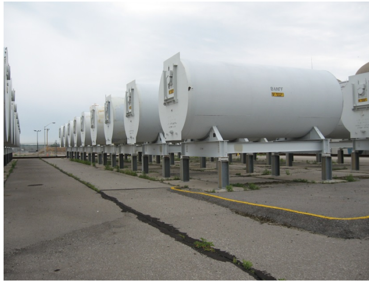
Figure H.1: Dry storage modules containing Pickering A (Units 1 to 4) retube waste at the Ontario Power Generation’s Pickering Waste Management Facility
