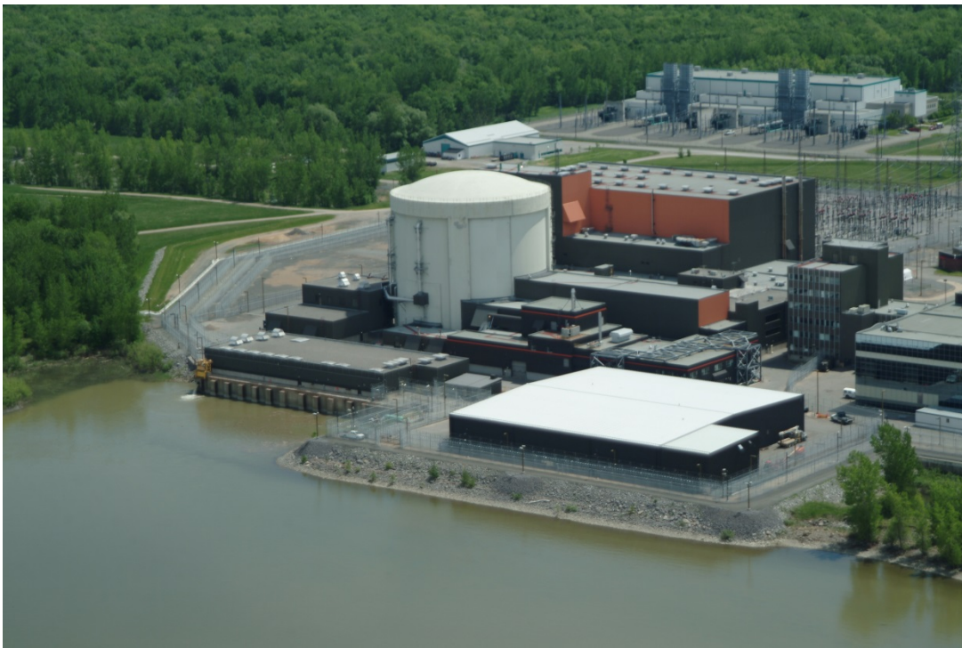
Figure 4.7: Gently-2 Nuclear Generating Station
