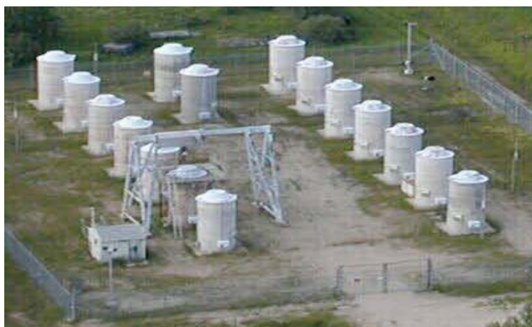
Figure 4.10 – Whiteshell Laboratories Concrete Canister Storage Facility (CCSF)
