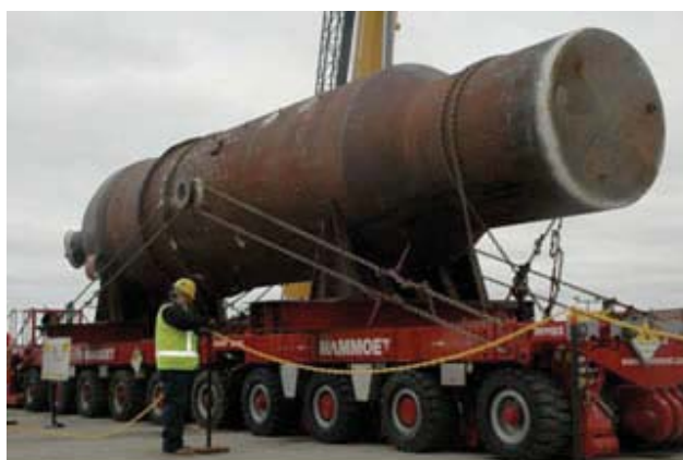
Figure H.2 – Steam generator being transported near the plant as part of the refurbishment
