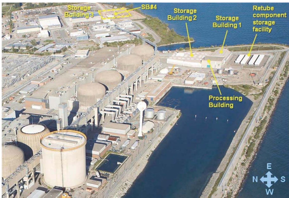
Figure 4.5 – PWMF I (Processing Building, Storage Buildings 1 and 2 and Retube Component Storage Facility) and PWMF II (Storage Building 3 and future Storage Building 4) area
