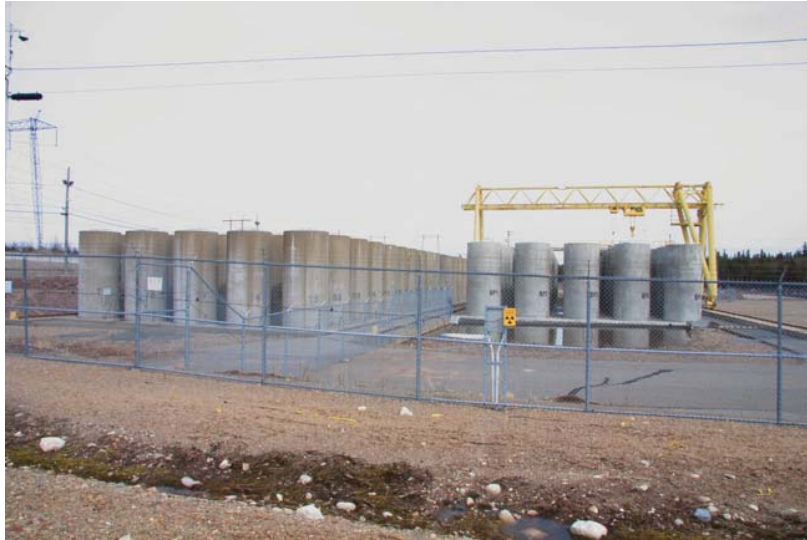
Figure 4.8 – Point Lepreau spent fuel dry storage area
