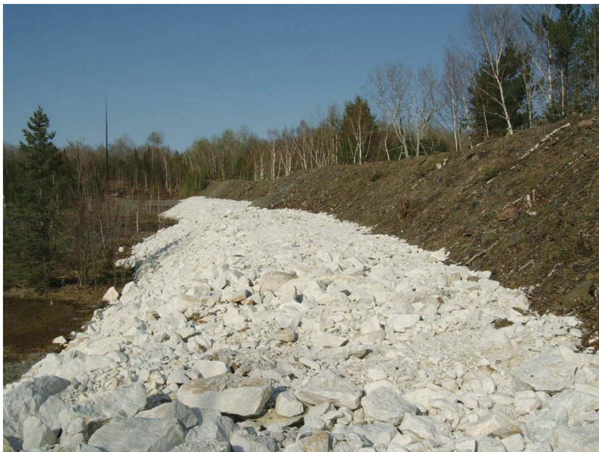
Figure 8.7 – Main tailings dam Dyno Mine site
