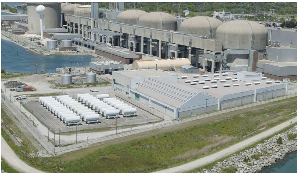
Figure 5.1 – Pickering Waste Management Facility, with RCSA (left) and spent fuel dry storage area (right)
