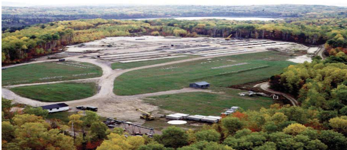
Figure 5.6 – Waste Management Area B at the CRL site
