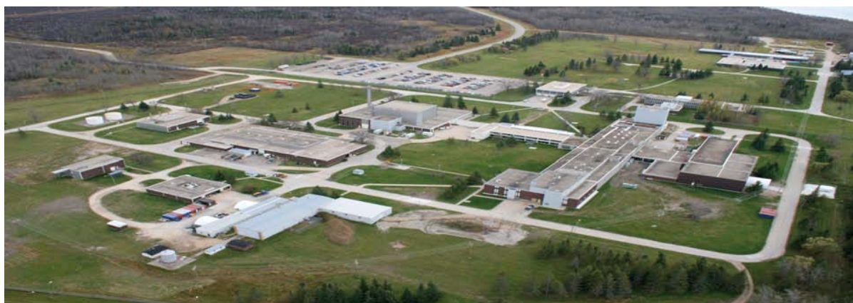
Figure 7.1 – Aerial view of Whiteshell Laboratories main site
