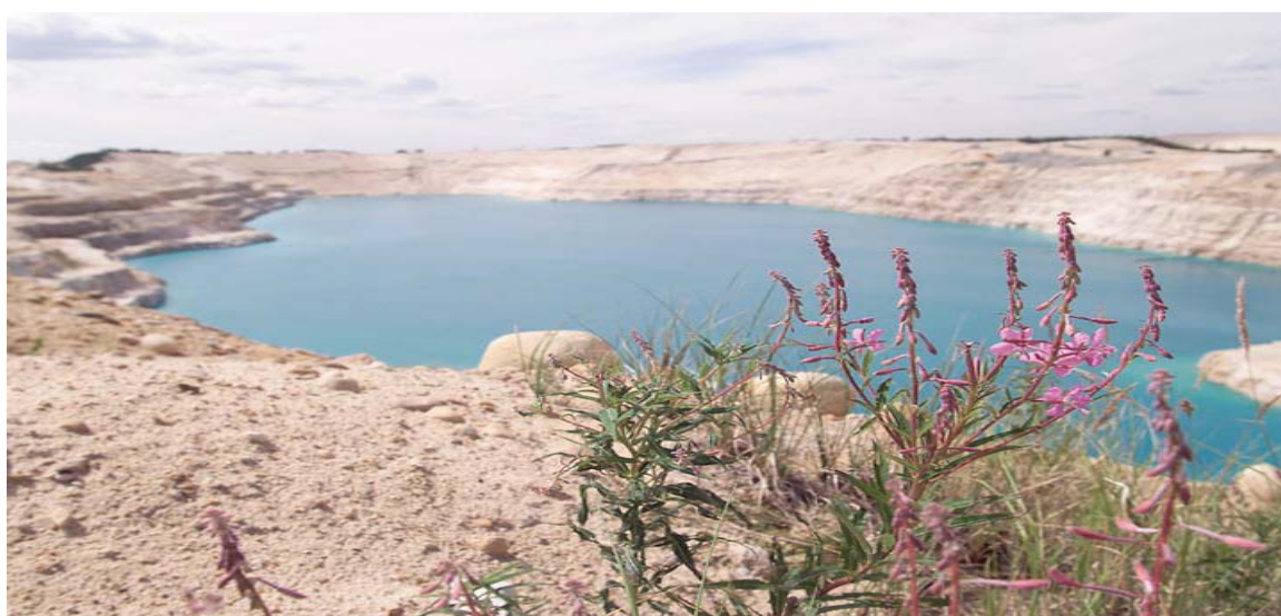
Figure 6.1 – Deilmann Tailings Management Facility at Key Lake
