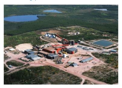
Figure 7.5: Cluff Lake mill area following decommissioning, but before vegetation became re-established
