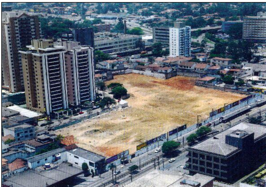
Figure F.10 - Clean area after USAM decommissioning work
