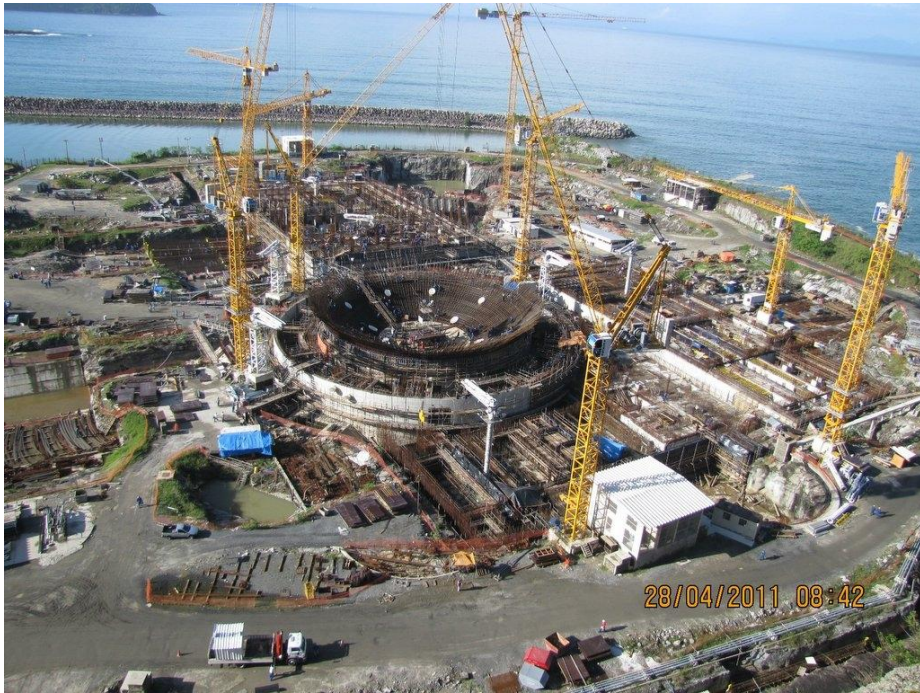
Figure D.1 - Angra-3 construction
