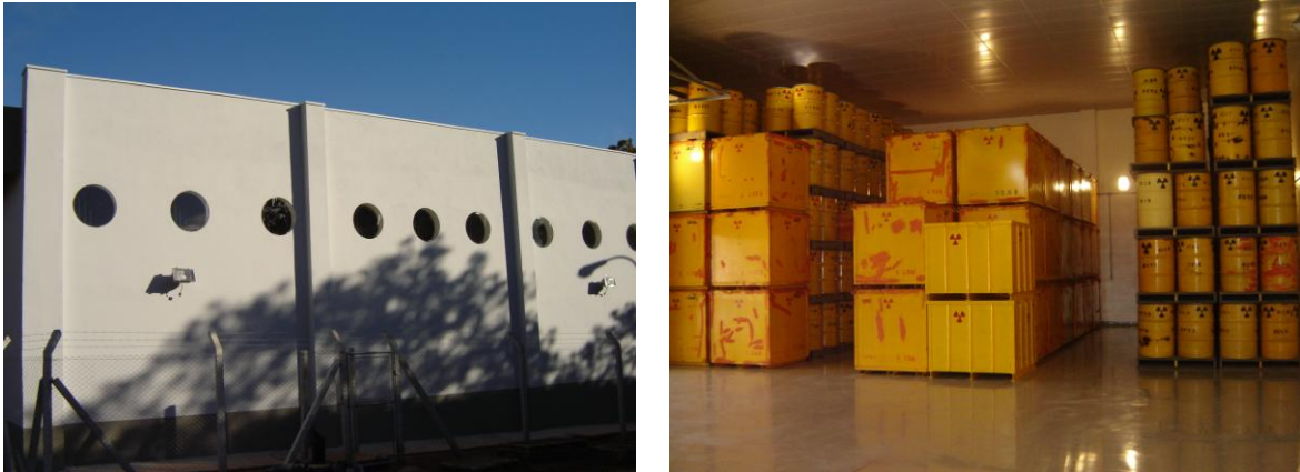
Figure k.1 -New radioactive waste storage (outside and inside view) at IPEN
