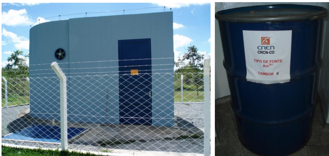
Figure D.3 - Interim storage facility at CRCN-CO
