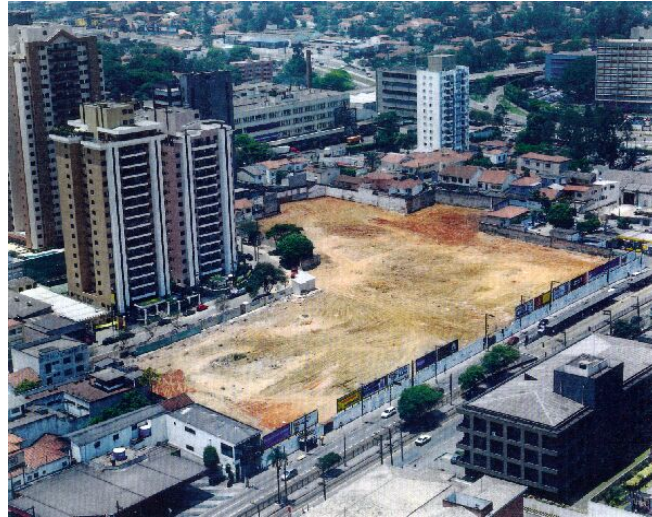
Figure F.7 –Clean area after USAM decommissioning work
