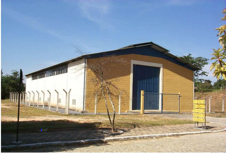
Fig. H.3. Intermediate Storage Building
