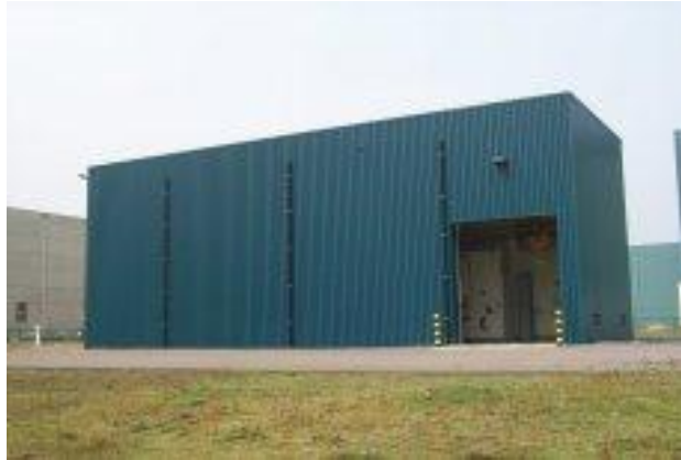
Figure 33: Exterior view of Building 156
