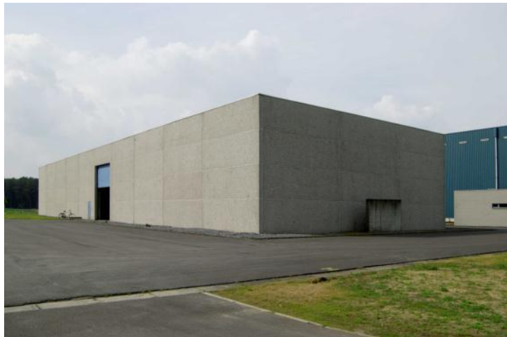
Figure 29: Exterior view of Building 150
