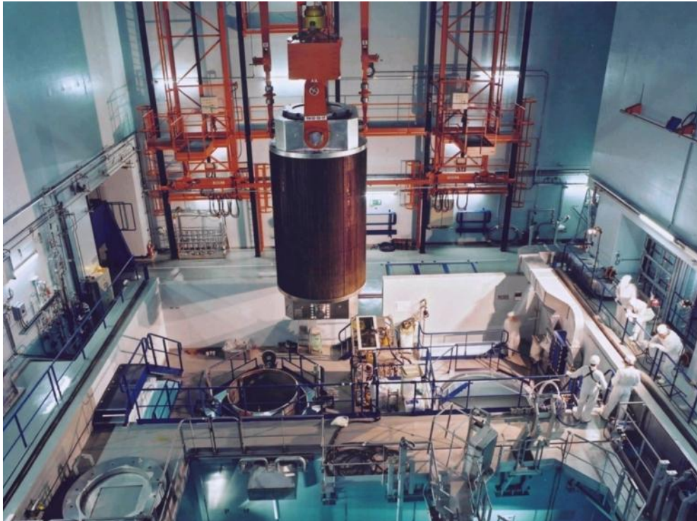
Figure 19: Intermediate Storage Building for Spent Fuel of Tihange
