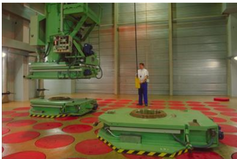
Figure 26: Hall above the storage bunkers
