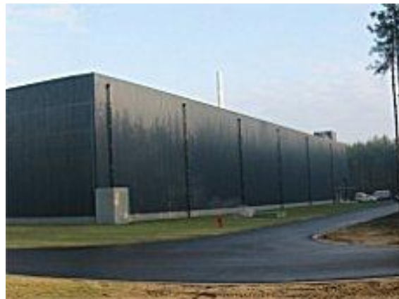
Figure 32: Exterior view of building 155
