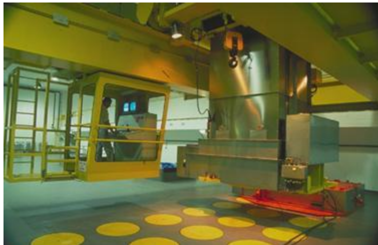
Figure 28: Interior view of building 136
