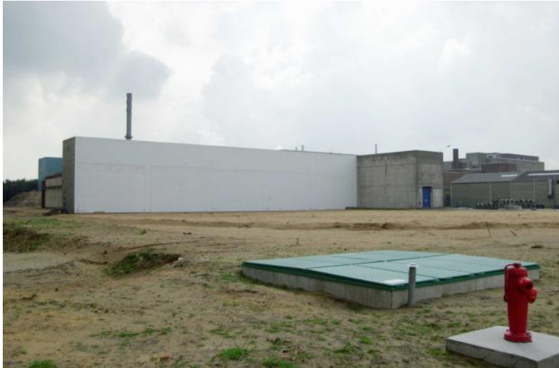
Figure 23: Exterior view of Building 127
