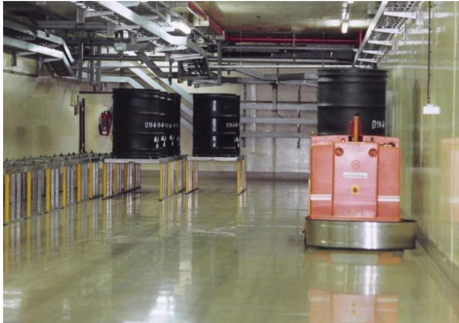
Figure 20: The WAB building (empty drums waiting for the next conditioning campaign)
