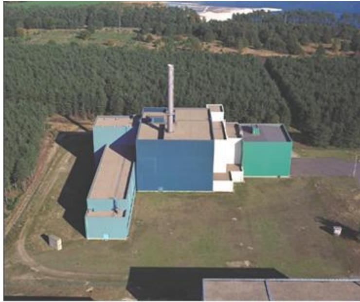
Figure 27: Exterior view of Building 136
