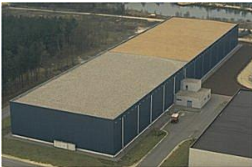
Figure 30: Exterior view of building 151
