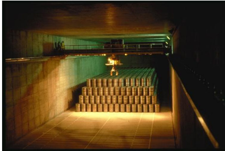
Figure 24: Interior view of a bunker in building 127
