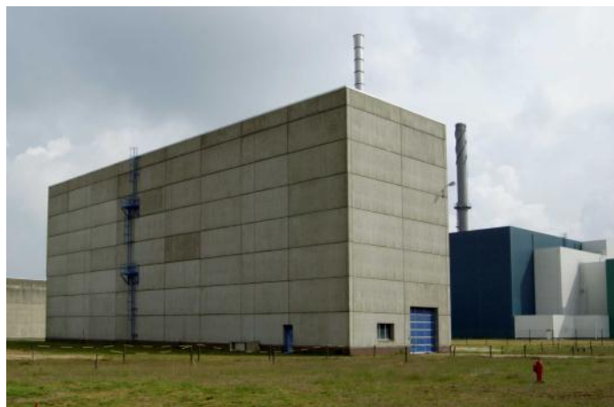
Figure 25: Exterior view of Building 129
