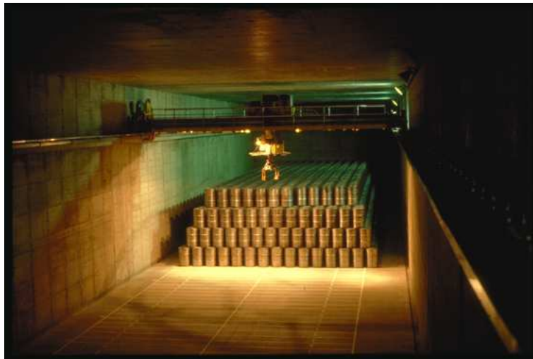
Interior view of a bunker in building 127
