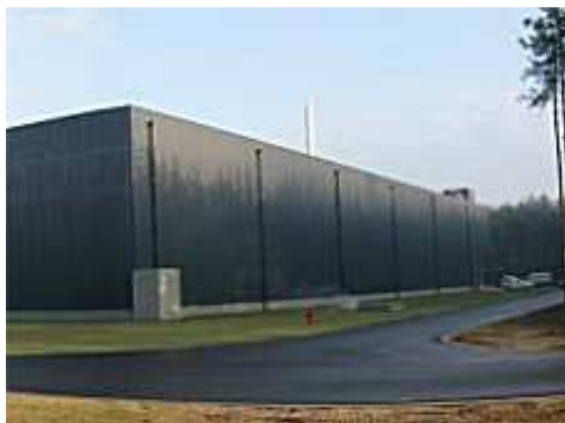
Exterior view of building 151
