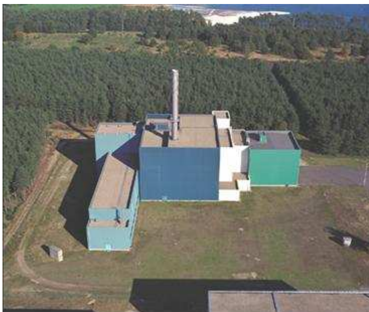
Exterior view of Building 136
