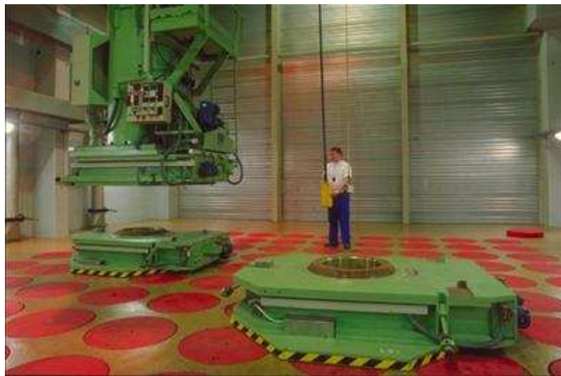
Hall above the storage bunkers
