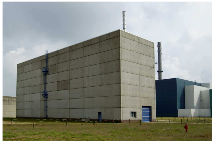
Exterior view of Building 129
