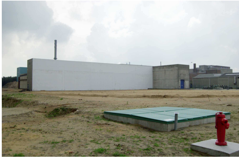
Exterior view of Building 127
