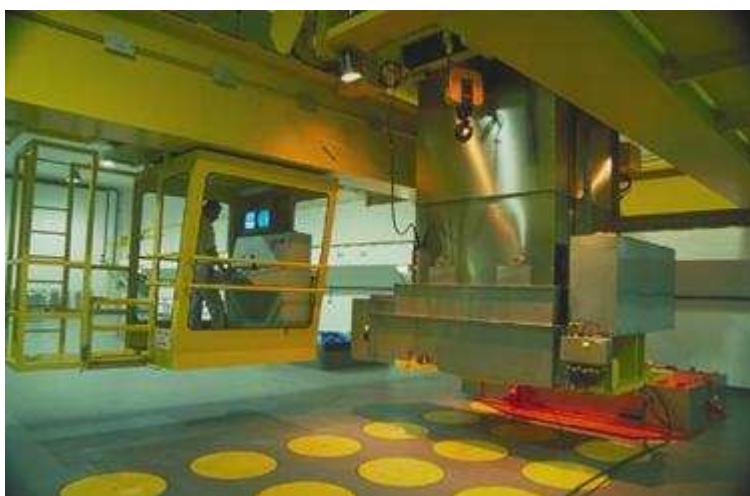
Interior view of building 136
