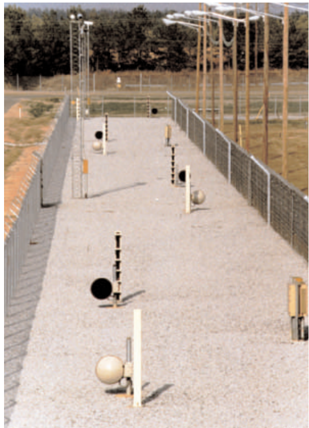
FIG. 1. An example of an exterior physical protection system for detecting and assessing intruders at a nuclear facility.
