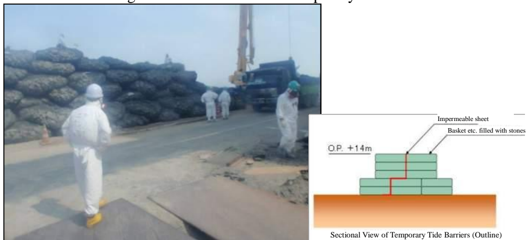
Fig. III-1-8 Installation of Temporary Tide Barriers
