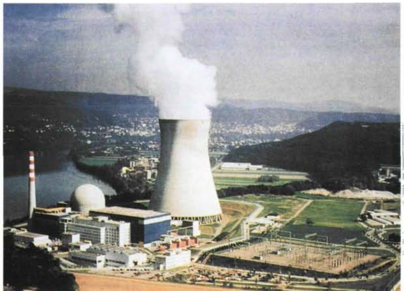
Leibstadt nuclear plant, Switzerland.
