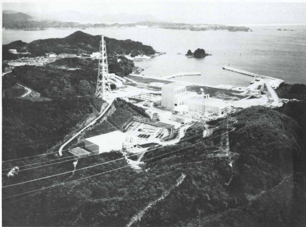
Onagawa nuclear plant, Japan.
