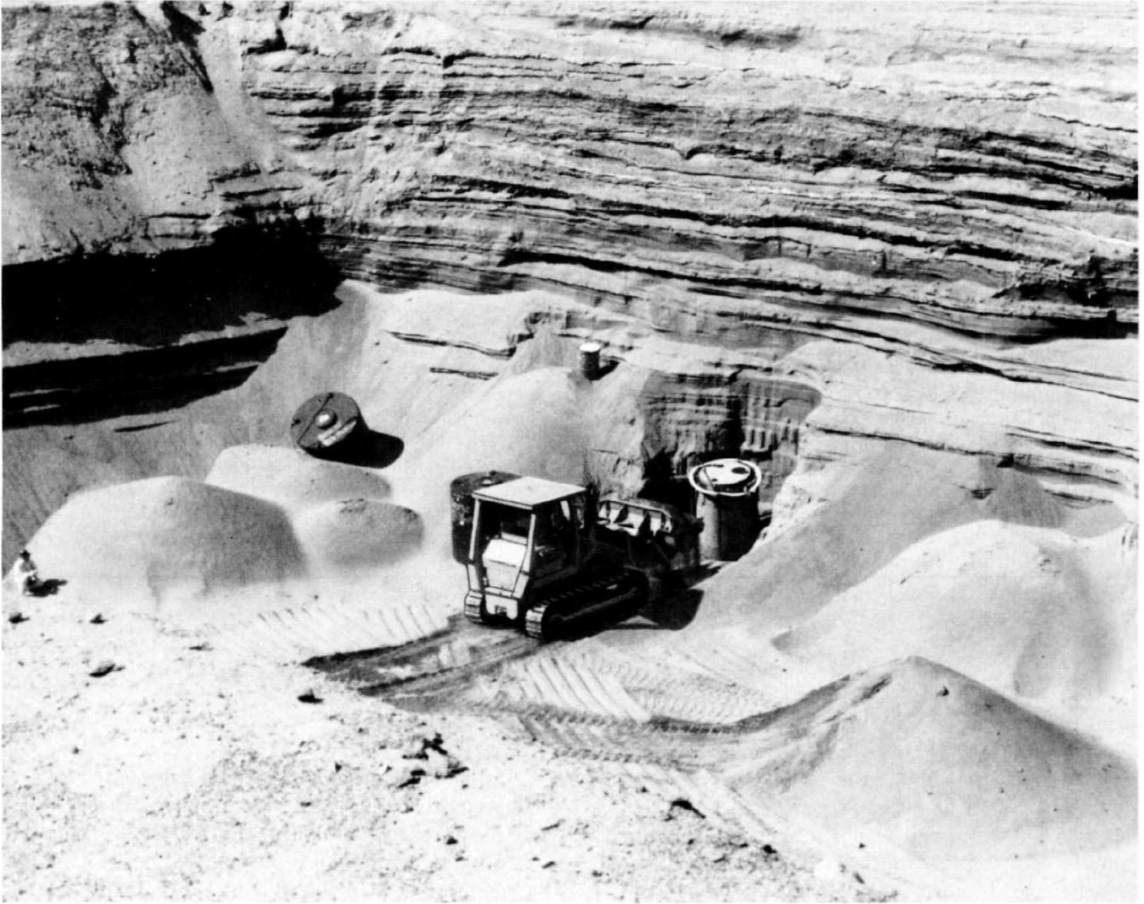
Containing an EPICOR-II prefilter, this demonstration "high integrity container" is being buried at the US Ecology disposal site for low-level radioactive waste.
