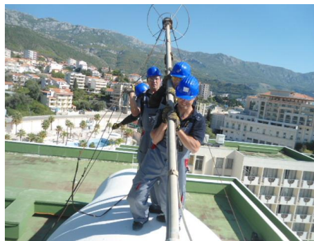
Picture 2: Removal of the radioactive lightning rod from the Hotel Mediteran in Bečići
