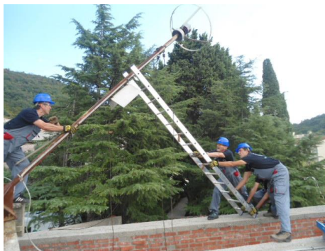
Picture 1: Removal of the radioactive lightning rod from the Hotel Castellastva in Petrovac
