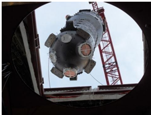
Figure 23 : SG Replacement at Doel 1
