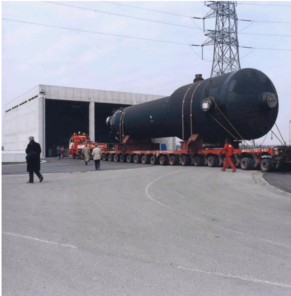
Figure 32 : Storage Building for Doel's Steam Generators
