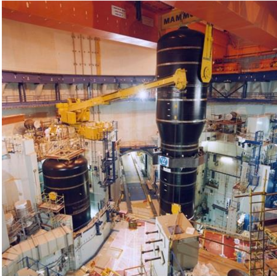
Figure 28 : Replacement of SGs of Tihange 3
