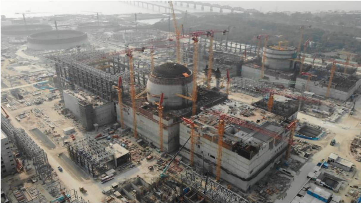
Figure 2: Construction of reactor building of Rooppur NPP Unit1 and 2
