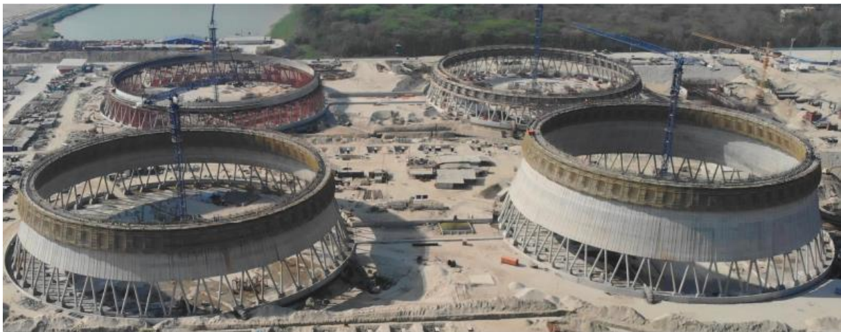
Figure 4: Construction of Cooling Towers – Rooppur NPP
