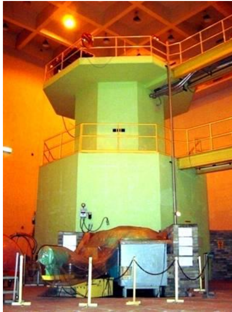
Figure 5: Reactor Hall of BAEC TRIGA Research Reactor (BTRR)
