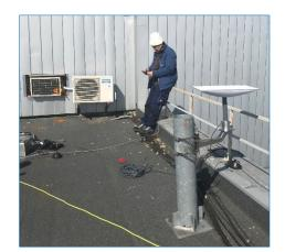
Figure 55: Enhancing the RDT Network: A Starlink satellite antenna was installed in Chornobyl in response to network disruptions caused by Ukrainian mobile network damage in the conflict's early stages (Q1 2022). The depicted Department staff member is setting up the antenna using a mobile app.
