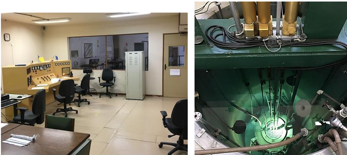
Figure 7 - IPR-R1 – Control Room and Reactor Pool
