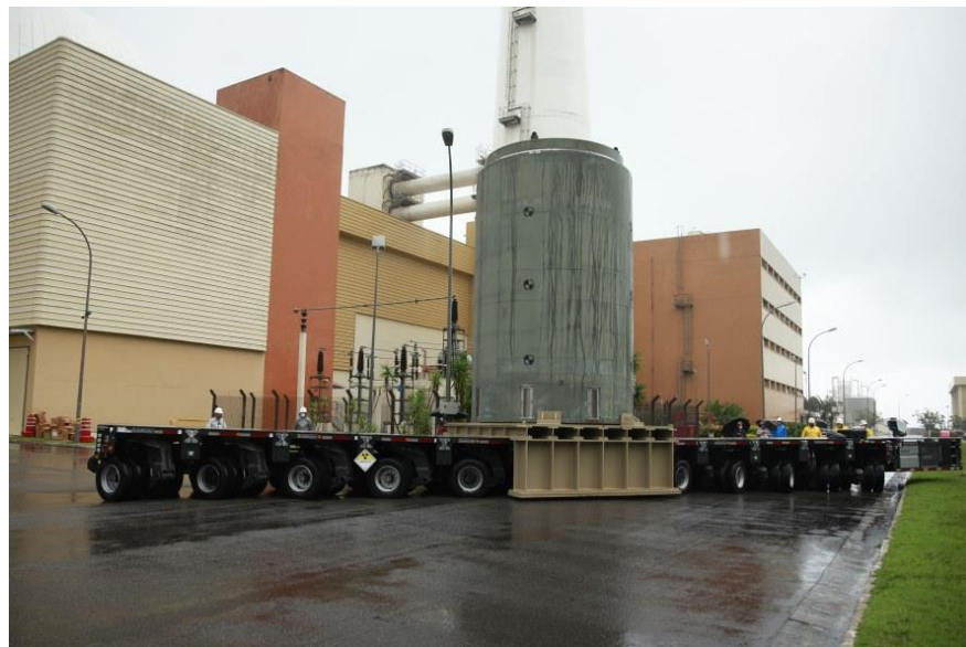
Figure 25 - Hi-Storm transfer to UAS (Credit: ABDAN)
