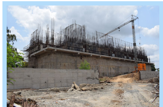
Construction activities of OESC at Kakrapar site
