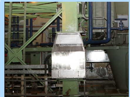
Passive Catalytic Recombiner Device
