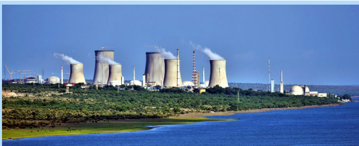
Rawatbhata Rajasthan Site
