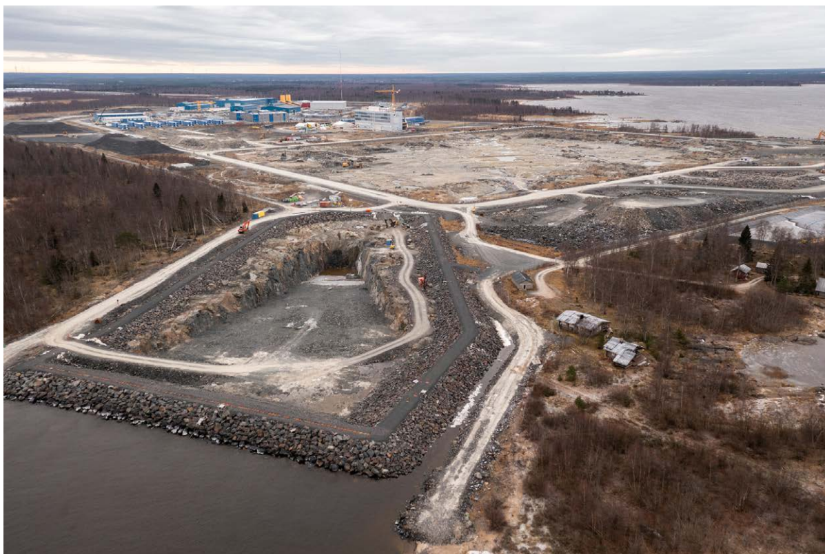
FIGURE 26. Hanhikivi site in Pyhäjoki: At front cooling water outlet channel with temporary dam and on the background NPP plant pit excavation down to -2m (FH1 November 2021). Source: Fennovoima.
