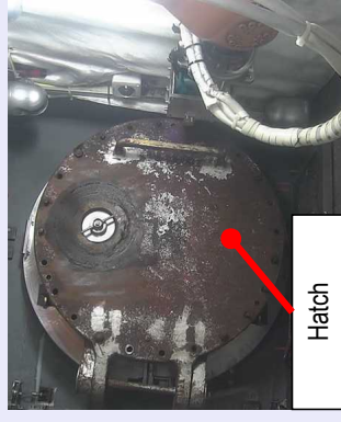
< Status of removal of bolts > (July 19, 2023)
