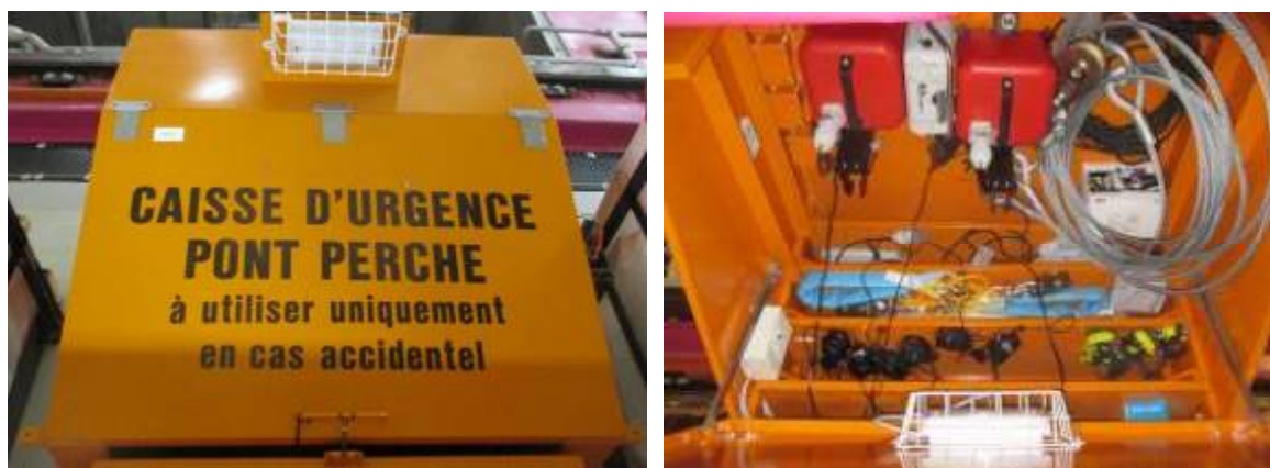
Fig.1 Post-Fukushima blackout box
