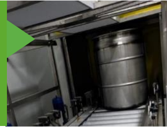
Radioactive waste treatment and conditioning
