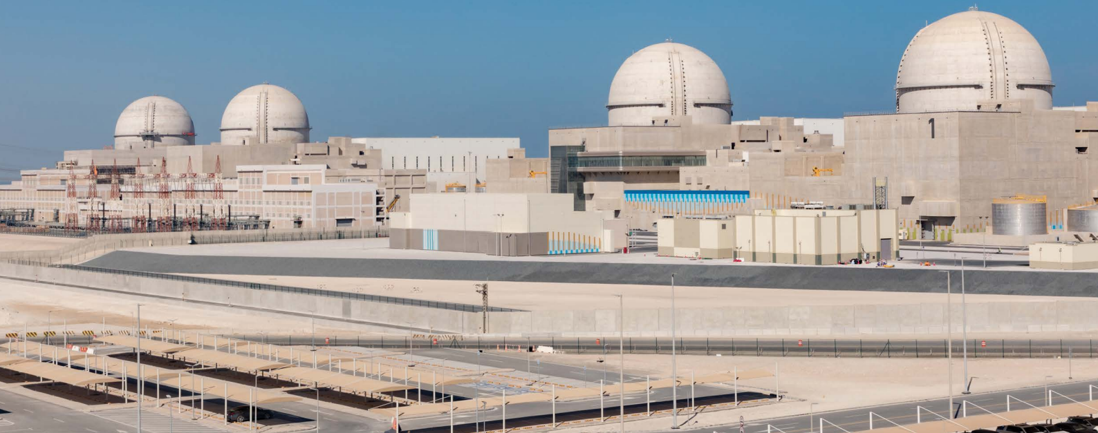
When fully operational, Barakah Nuclear Power Plant in the United Arab Emirates will meet almost 25 per cent of the country's electricity demand, making a significant impact on efforts to fight climate change. (Photo: ENEC)
