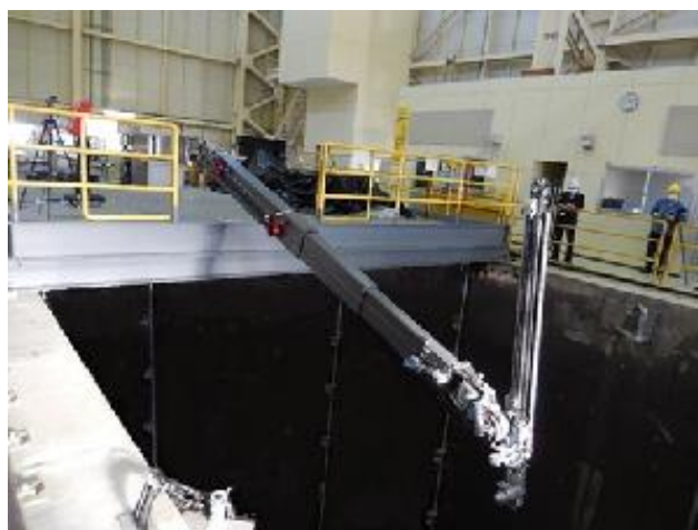
Image: Equipment for the Unit 2 trial fuel debris retrieval
