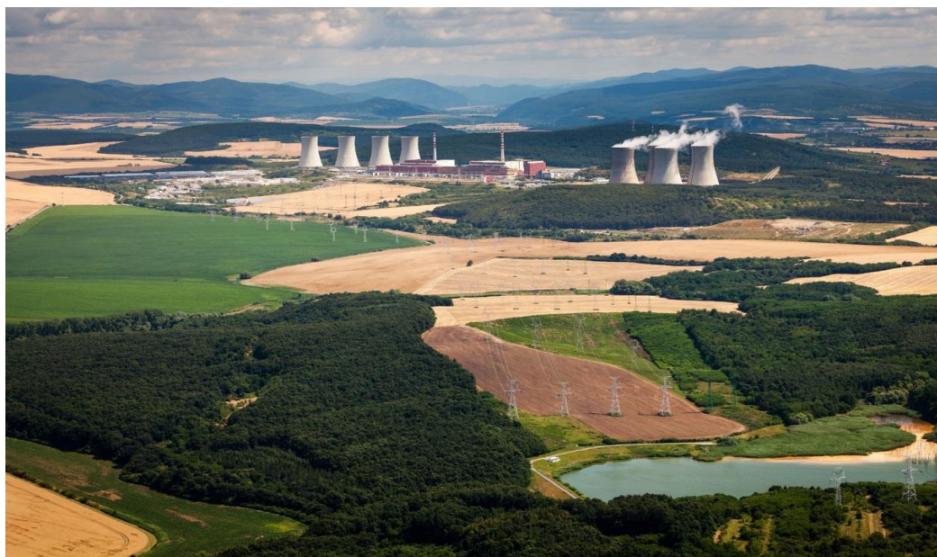
Fig. 6 Nuclear Power Plant Mochovce site
