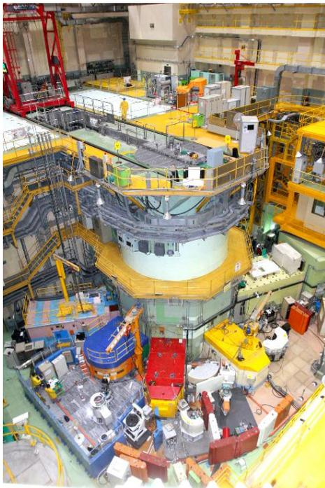
HANARO complex is composed of the HANARO research reactor and ancillary facilities such as the Cold Neutron Research Facility (CNRF), Radioisotope Production Facility (RIPF), and Irradiated Material Examination Facility (IMEF). The HANARO and ancillary facilities were designated as an ICERR by the IAEA in 2019.
