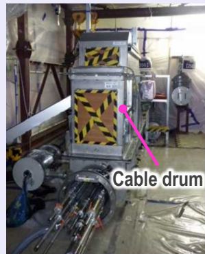
<Installation of equipment>
