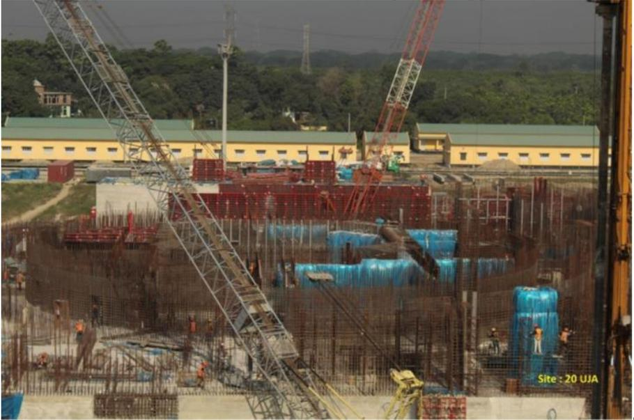
Figure 3: Construction of reactor building of Rooppur NPP Unit 2
