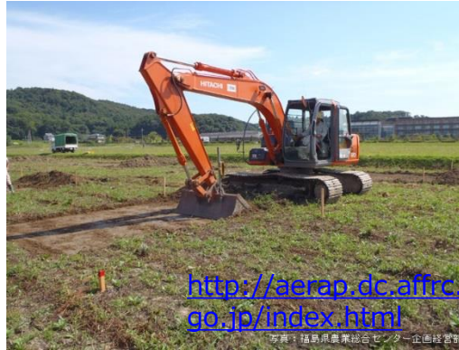
Removal of surface soil
