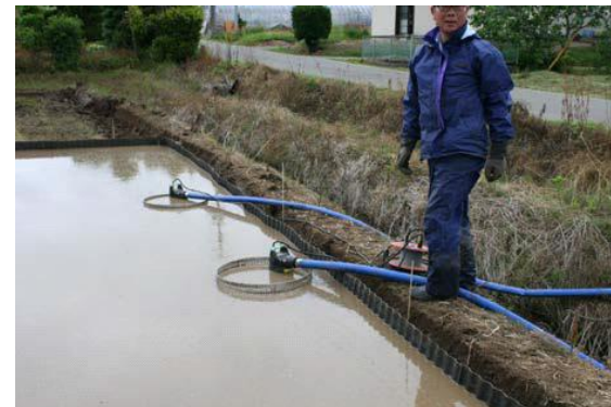
3. Removal of soil suspension from the paddy by pumping
