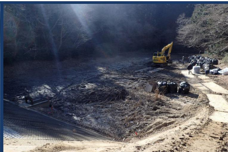
Sediment removal from irrigation
