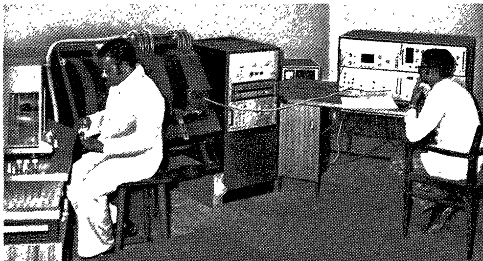
Analysis of the oil content of oilseeds is carried out with a nuclear magnetic resonance (NMR) machine at the Institute.
