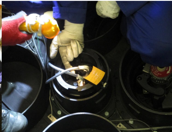
Trainees checking control rod cables – simulated contamination control area
