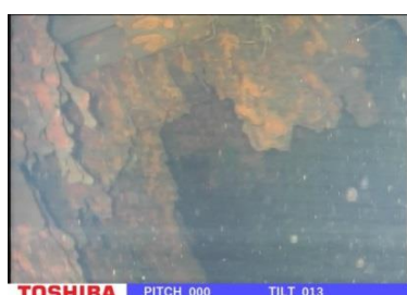
bottom of CRD housing
