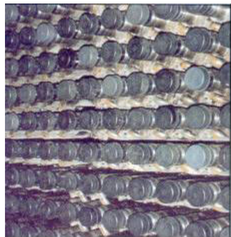
Figure 1: End fitting plugs and fuel bundles.
