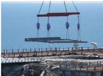
Installing shields on the operating floor
