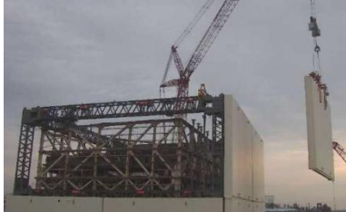
Removal of wall panels
