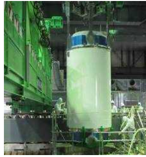
Storage of removed fuel
