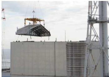
Removal of roof panels
