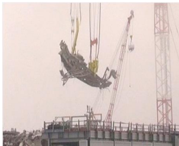
Removal of FHM
