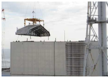
Removal of roof panels
