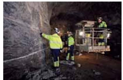
*The host rock is carefully studied to ensure its suitability for final disposal of spent fuel. At the Finnish disposal site, the excavation of the access tunnel reached the final disposal depth 420 metres in 2010.*
