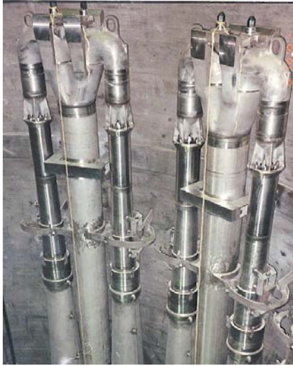
Jet Pumps Assembly-Construction
