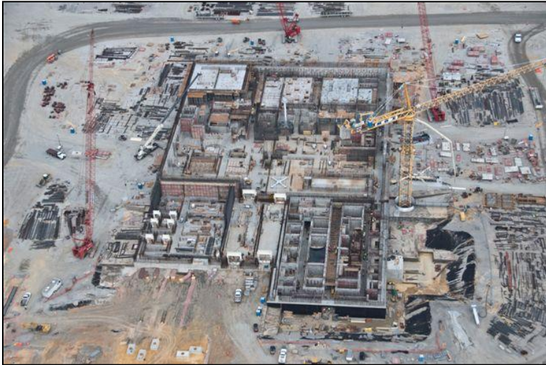
MOX Plant in construction (Savannah River)
