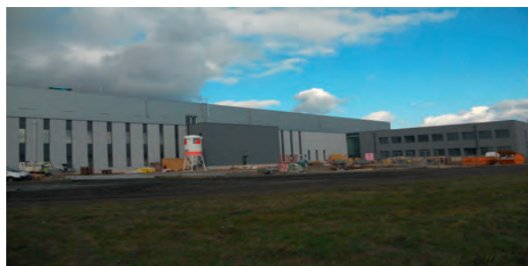
FIG. 3. View of the construction activities for the Nuclear Material Laboratory in Seibersdorf, Austria, November 2012.
