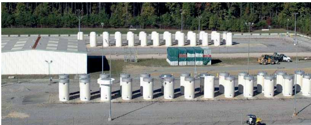
FIG. 4. The Independent Spent Fuel Storage Installation at the Surry Nuclear Power Plant in Virginia, USA, an at-reactor dry storage cask facility.
