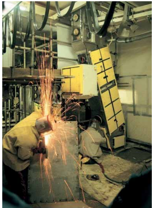
FIG. 1. Decommissioning of a glove box in a fuel fabrication facility.
