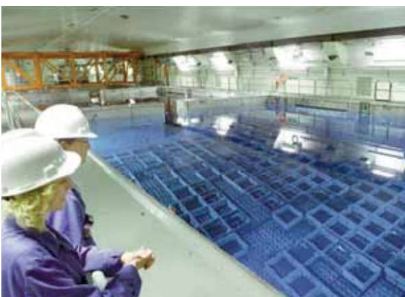
FIG. 3. The Central Interim Storage Facility for Spent Nuclear Fuel (CLAB) at Oskarshamn, Sweden, an away from the reactor underground wet storage pool facility.
